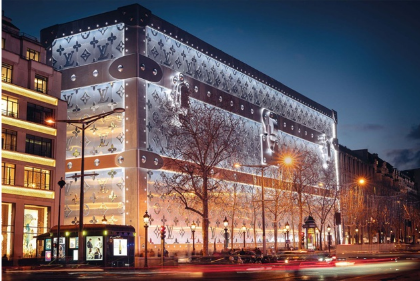
103 - Louis Vuitton trunk installation Temporary construction enclosure
